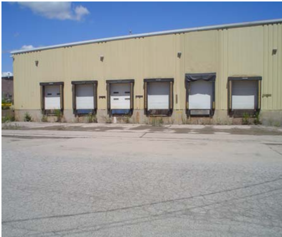
Main Building Shipping Area
